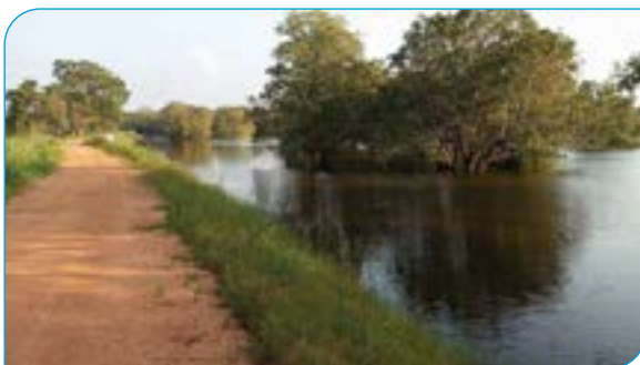
Fig. 2 Galkande Wewa, located in Sri Lanka's Anuradhapura District, was rehabilitated in 2024. The restored tank now provides reliable water for 20 farming families and is able to retain water even through the end of the dry season [Attribution: SARP]
